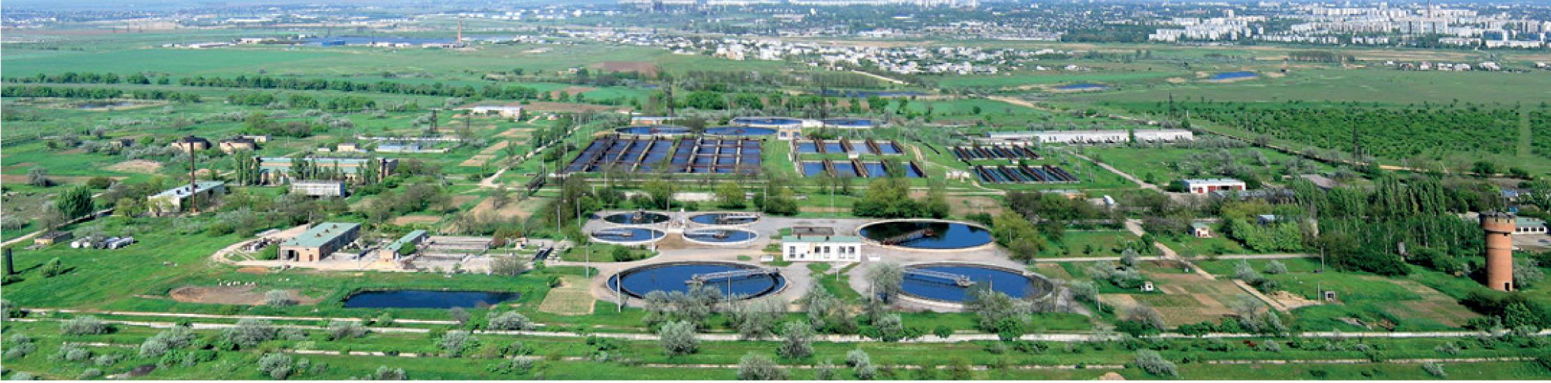
The capacity of the facility is 250,000 m3 per day Actual 43 thousand m3 per day Energy consumption 12 thousand kWh per day Specific energy consumption 0.28 kW/m3 The area of MOS is 85.31 ha 41.2% Efficiency of mechanical cleaning Efficiency of biological cleaning 91.6%
