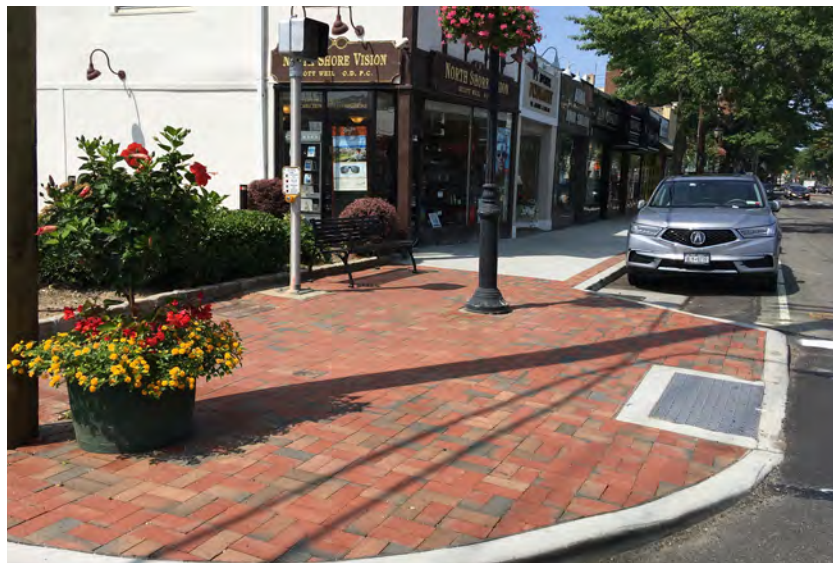
ADA Compliant brick curb extension with planters.
