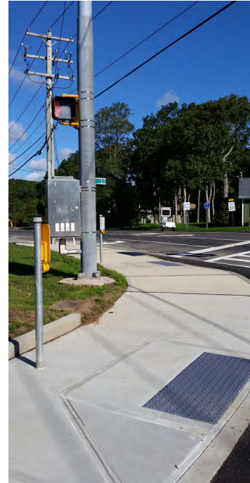
Top Left: ADA compliant pedestrian ramp with push button and new sidewalks.
