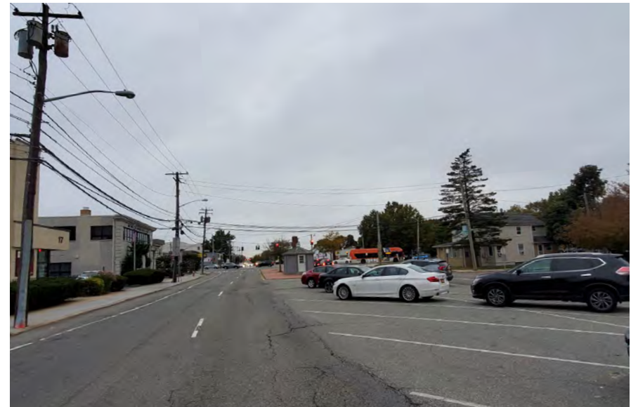
John St median from street level.
