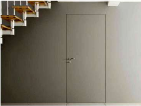
The door leaf on the entrance side is laminated MDF *, similar to the facade of the built-in wardrobe.
