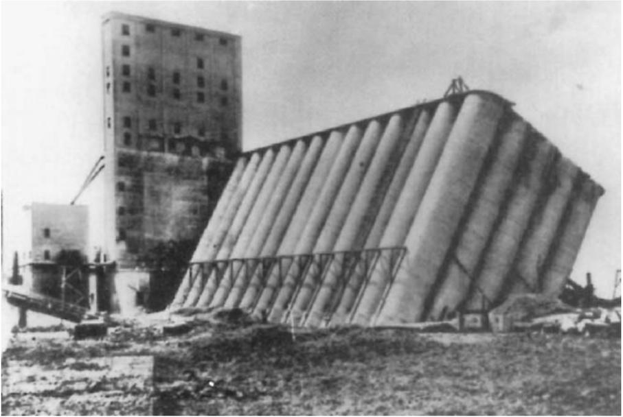
FIGURE 6.27 Transcona grain elevator bearing capacity failure.
