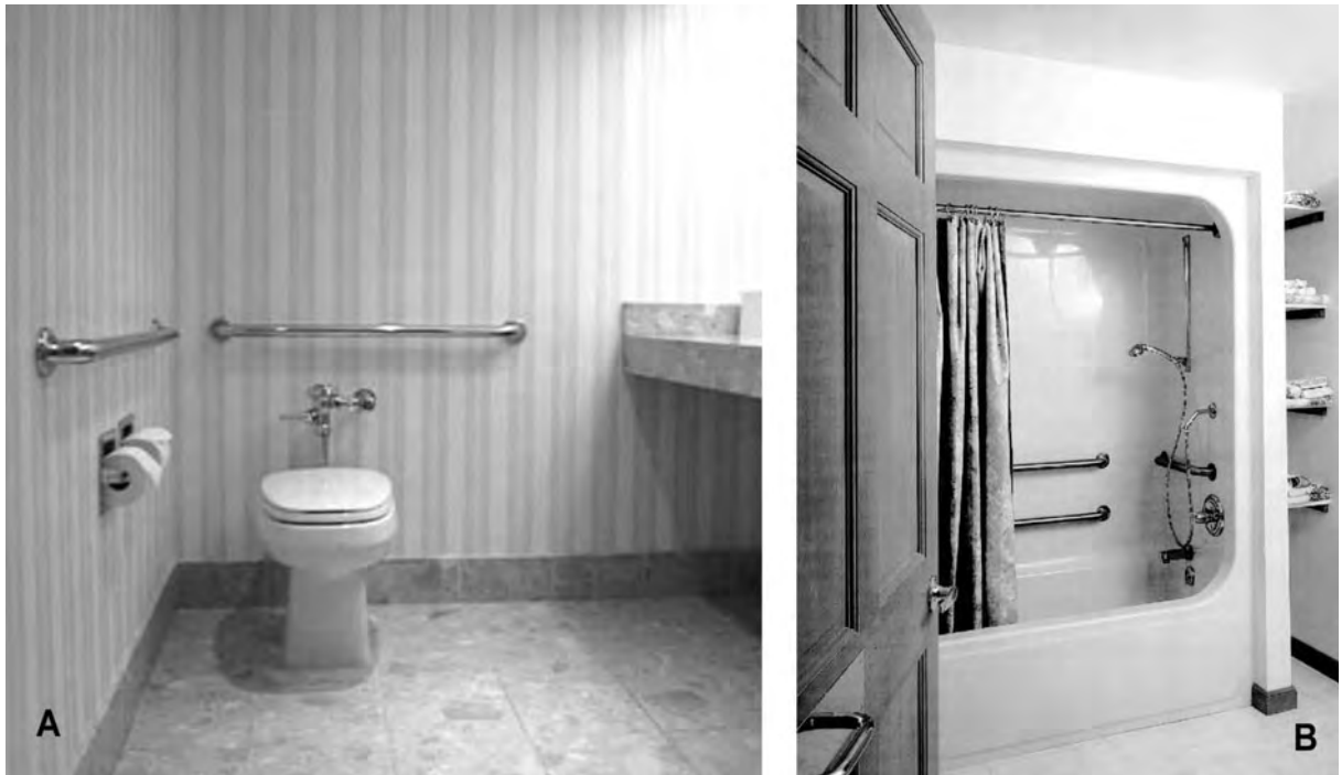
Figure 11.10 A. A typical accessible bathroom in a senior living complex in Maryland. B. A prefabricated shower unit with strong grab bars (source: Charles A. Riley II).
