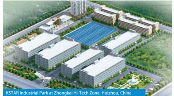
KSTAR Industrial Park at Zhongkai Hi-Tech Zone, Huizhou, China
