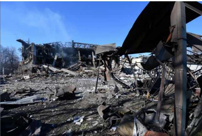
Destroyed airport «Dnipro» and infrastructure nearby
