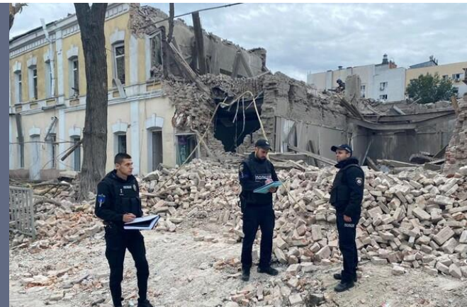
Destruction of the historical buildings of the city center
