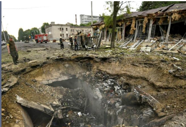
The enemy missile destroyed the city's infrastructure and buildings. Several people died
