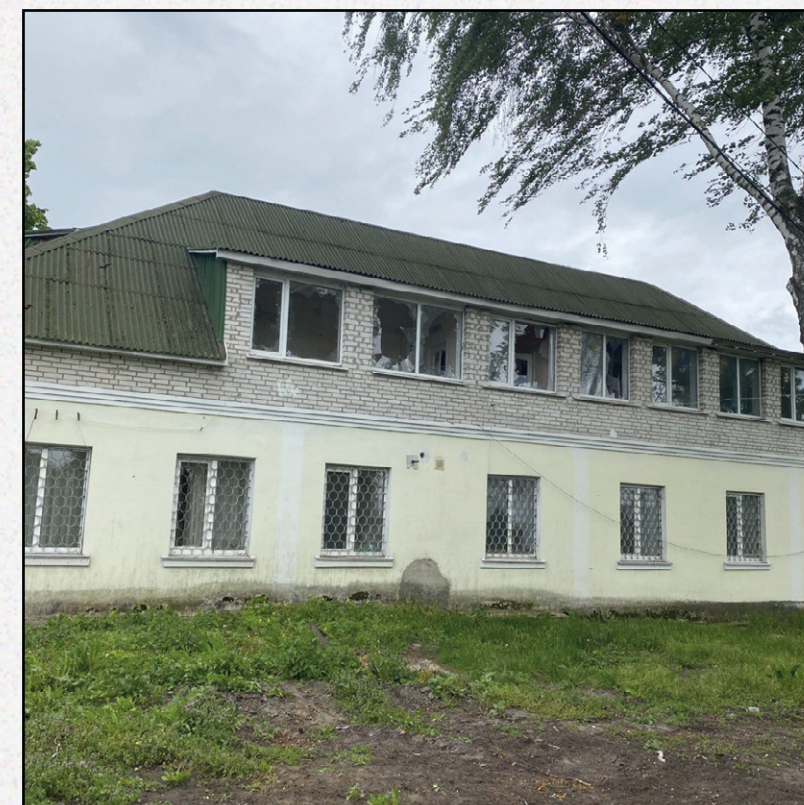
Administrative service center
