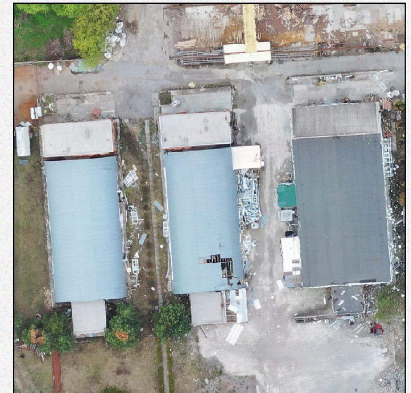
Warehouse complex MAKARIV
