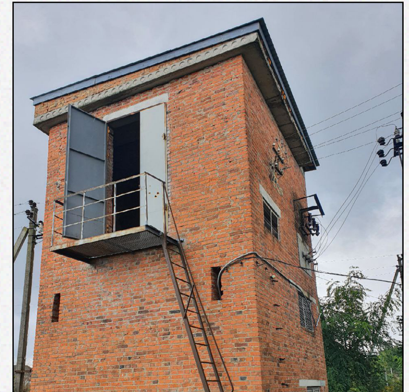
Building of communal economy
