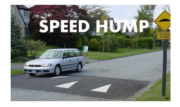
**Speed Humps** Used where AADT is <3500\* / posted speed <30mph
