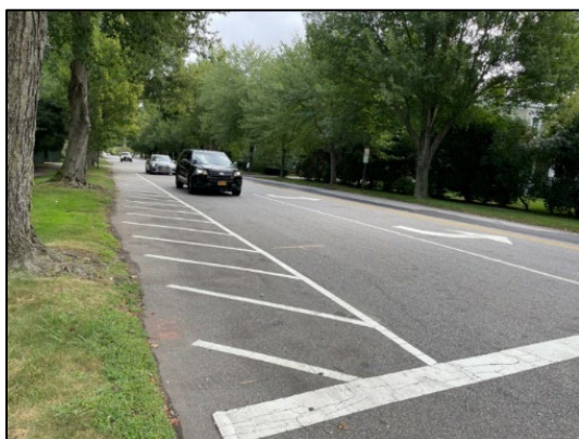
Figure 19: Striping, or pavement markings, can be used to narrow roadways
