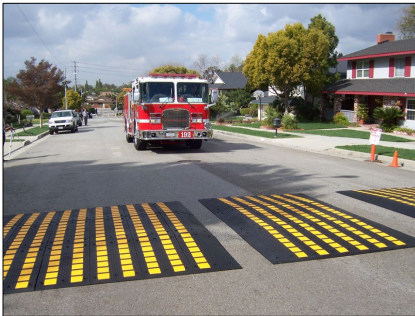
Figure 21: Speed cushions allow emergency services vehicles to pass without reducing speed
