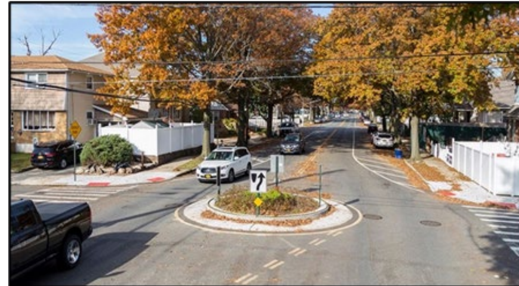
Figure 28: Traffic circles can be built with permanent or mountable materials to slow vehicles approaches at intersections
