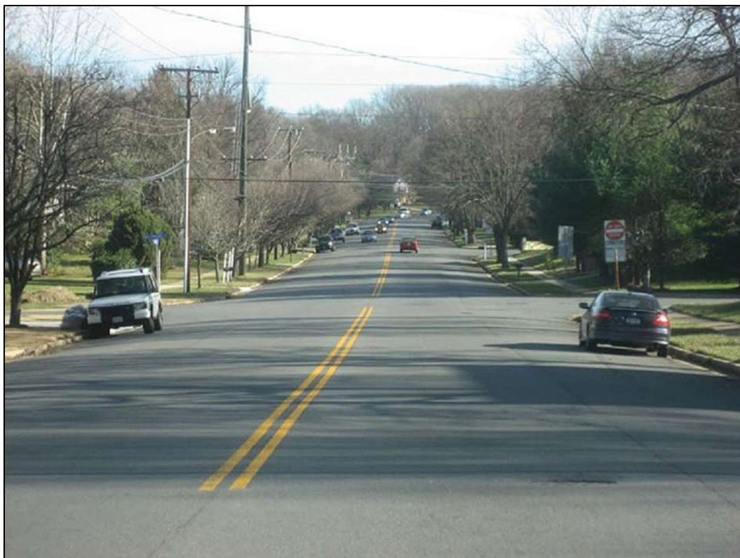
Figure 29: Wide two-lane street before a road diet, with excess vehicle capacity
