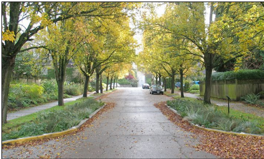
Figure 23: Chokers can be used to narrow the street by extending one or both curbs
