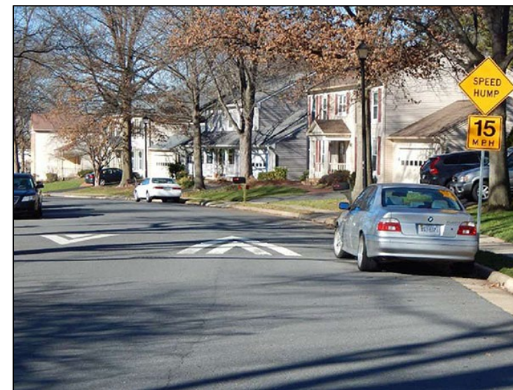
Figure 20: Speed humps are effective at slowing traffic
