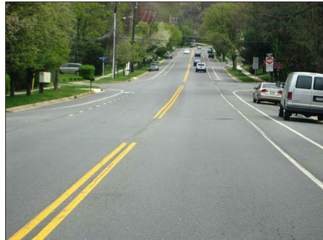
Figure 30: The same street as shown in Figure 29 after implementation of a road diet with standard bike lanes
