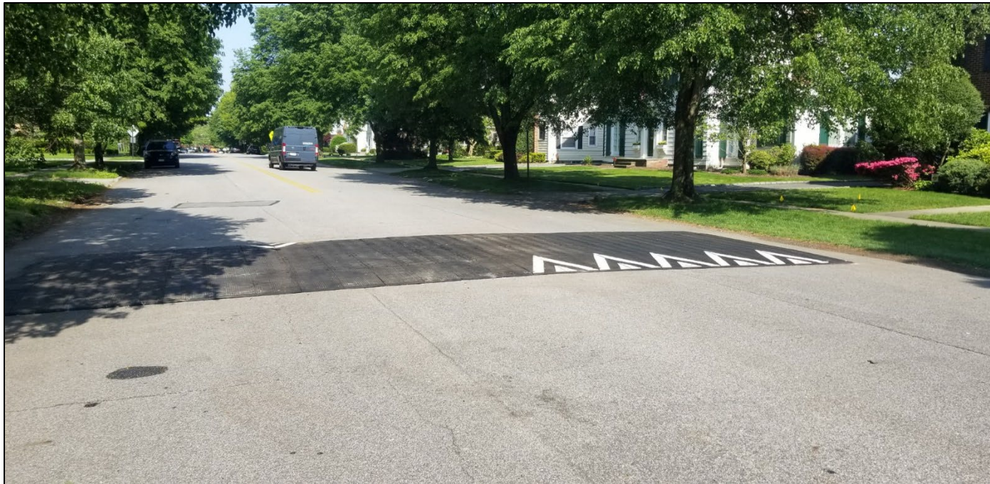
Figure 44: Speed hump constructed with temporary materials and installed on 4th St in Garden City in May 2023
