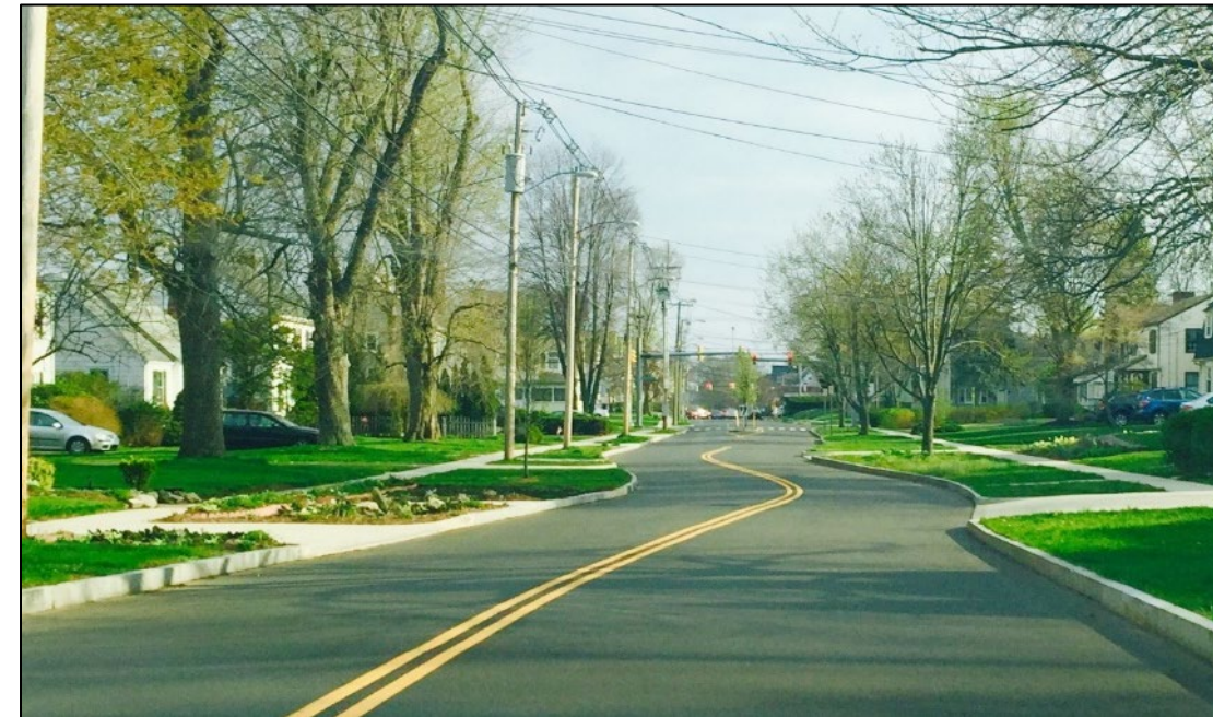
Figure 24: Chicanes change the alignment of the roadway which encourages slower speeds to navigate.
