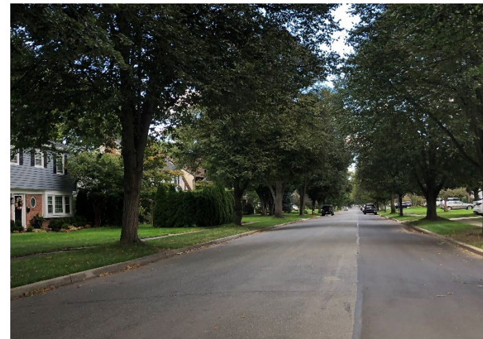
Figure 6. Many of the streets are over 30 feet and have little or no on-street parking, which creates two very wide travel lanes.
