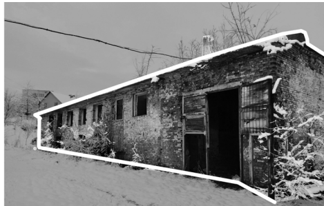
Figure. 46. Photo of the annex utility building of the boiler room Source: local activist O.Tsiupur
