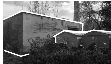
Figure. 62. Existing illegal garages on the territory Source: Ro3kvit
