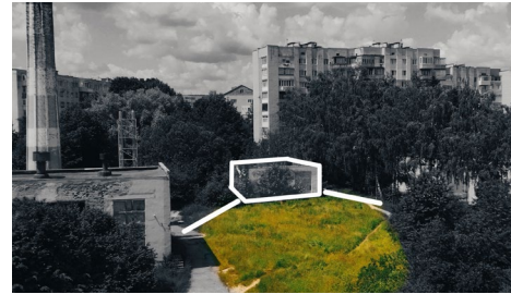
Figure. 58. Photo of the boiler room and its auxiliary building Source: Ro3kvit
