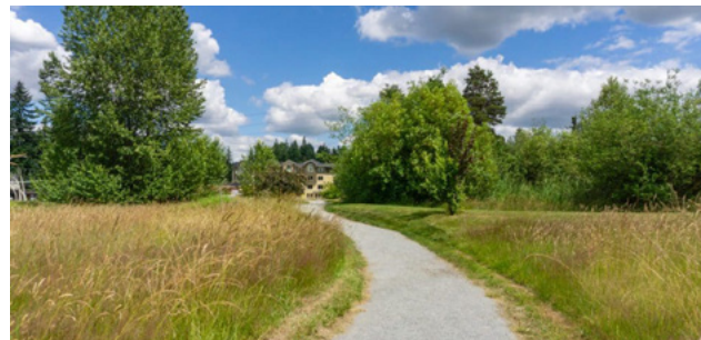
Figure 92. Compacted mineral path surface Source: www.wa-rock.com
