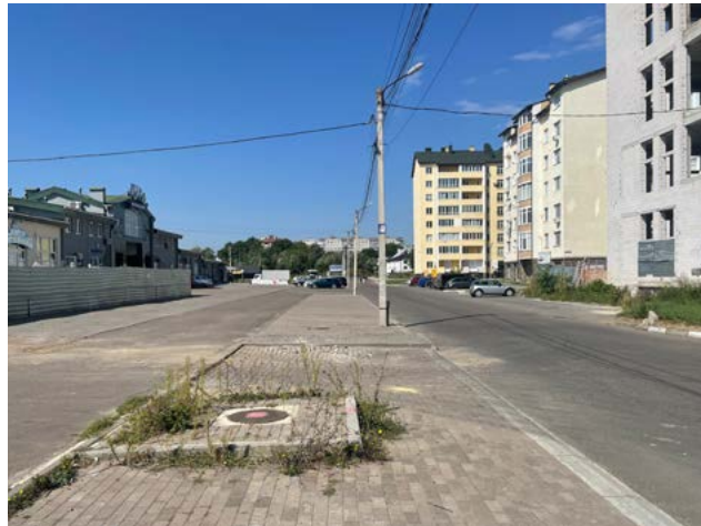
Figure. 18 Image 2 on the photo of the planning area Source: Ro3kvit
