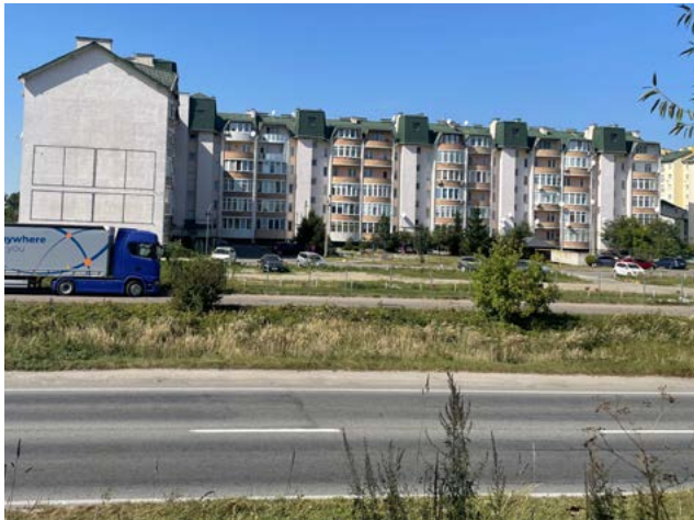
Figure. 17 Image 1 on the photo of the planning area Source: Ro3kvit
