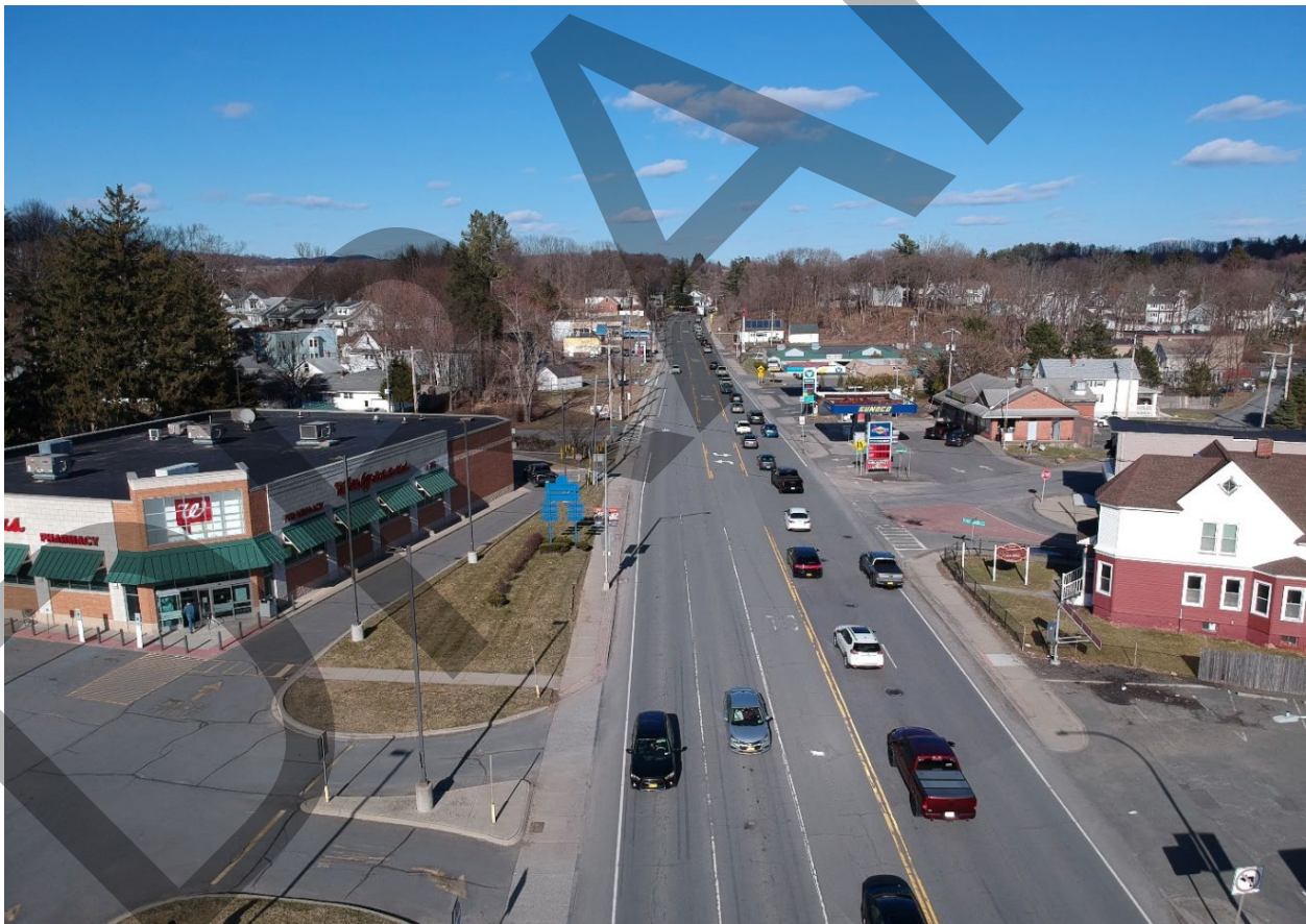
IMAGE 1.1: TYPICAL CONGESTION EAST OF N. LAKE AVENUE
