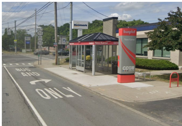
FIGURE 3.8: BUS TURNOUT EXAMPLE
