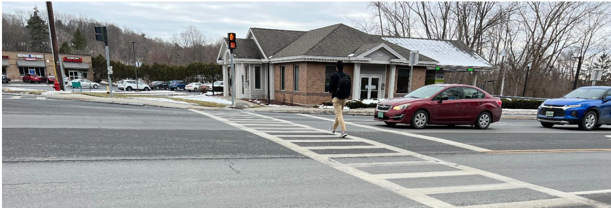
IMAGE 2.2 –EXAMPLE OF PEDESTRIAN CROSSING AT A MARKED CROSSWALK ON HOOSICK ROAD
