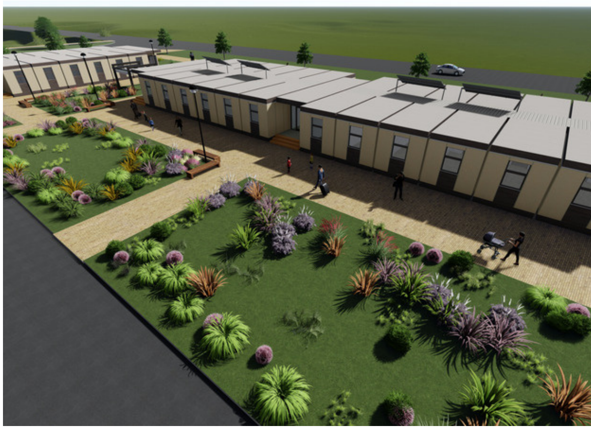
CONSTRUCTION OF A MODULAR TOWN FOR INTERNALLY DISPLACED PERSONS
