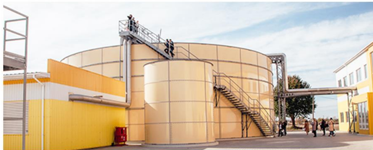
RECONSTRUCTION OF SEWAGE TREATMENT FACILITIES
