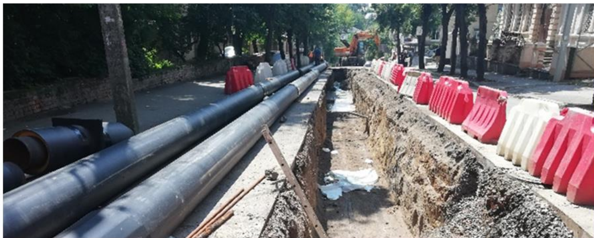
RECONSTRUCTION OF HEATING NETWORK
