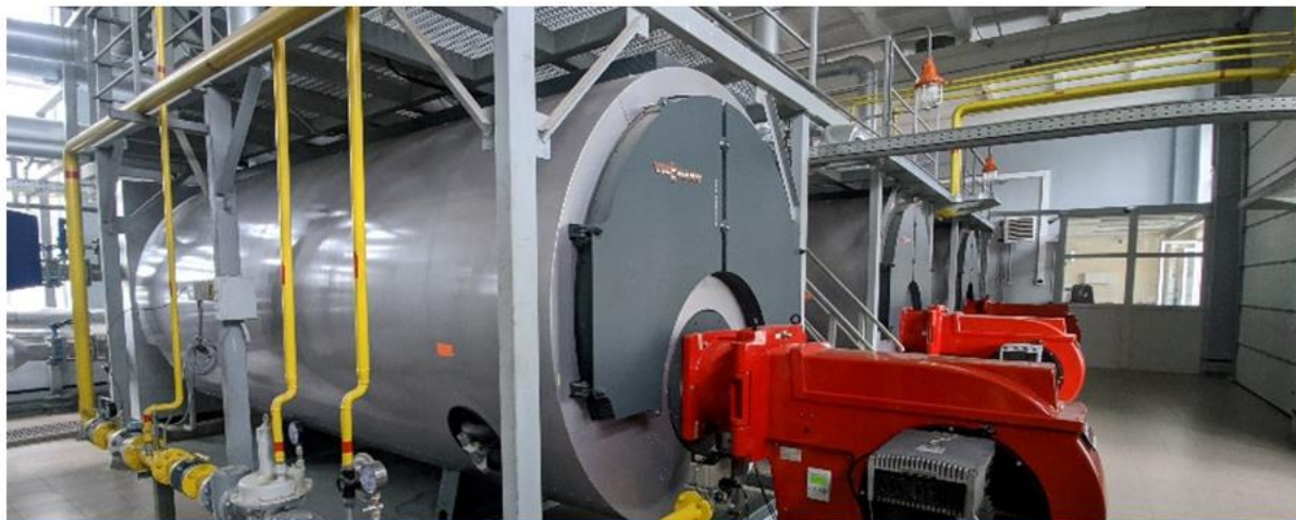
RECONSTRUCTION OF BOILER HOUSE
