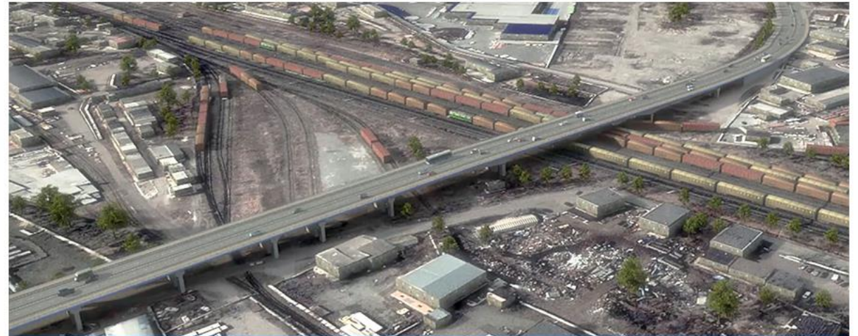
CONSTRUCTION OF A ROAD OVERPASS OVER THE RAILROAD TRACKS
