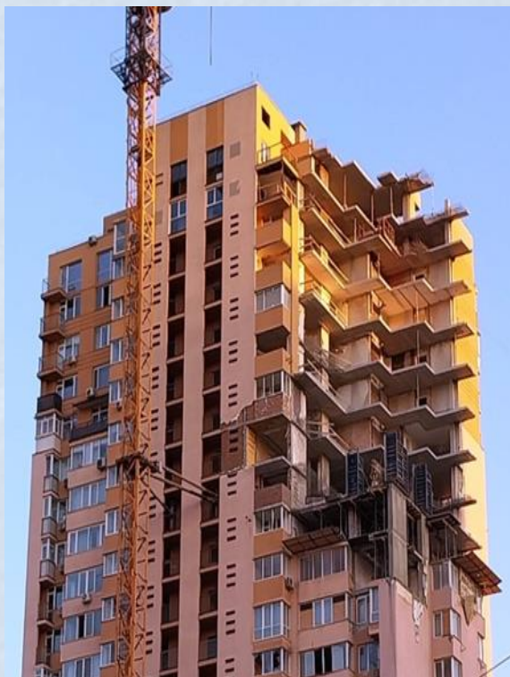
September 08, 2022 (concreting of poles and floor slabs)
