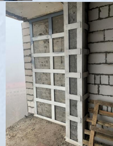
Installation of reinforcement to wall panels
