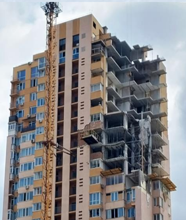
August 19, 2022 (dismantling during temporary unfastening)
