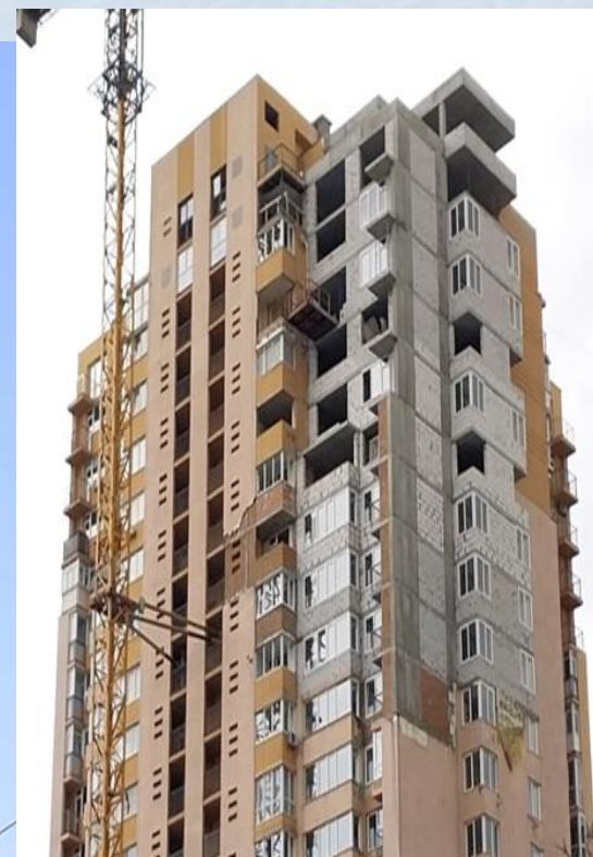
October 27, 2022 (reconstruction of walls and windows)
