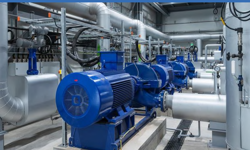
Reconstruction of Sewage Pumping Station IA
