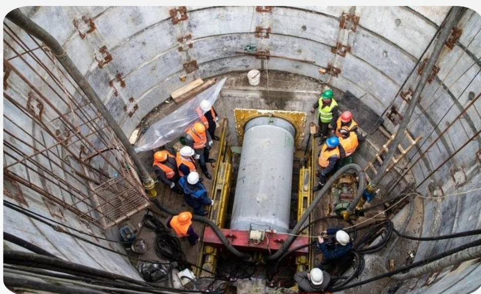
Reconstruction of the section of the main sewage collector - 1 932 616 EUR
