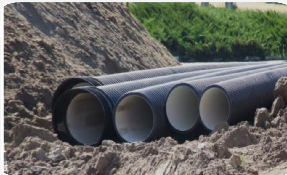
Reconstruction of the section of the main sewage collector - 1 064 275 EUR
