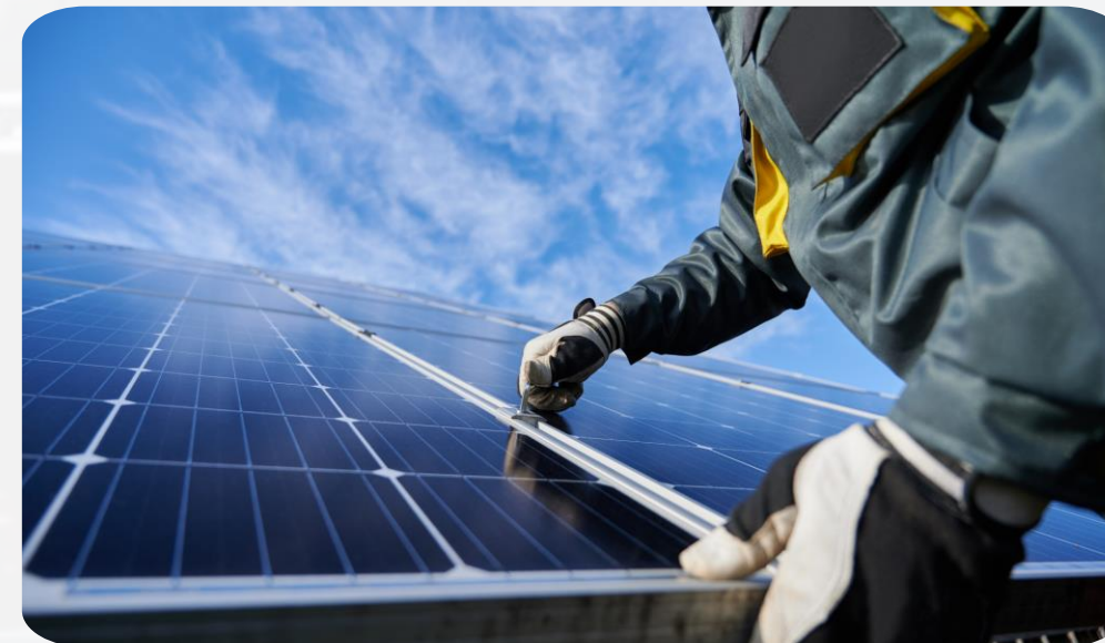
Solar power station at the reserve water intake "Vilshanka" - 932 398 EUR
