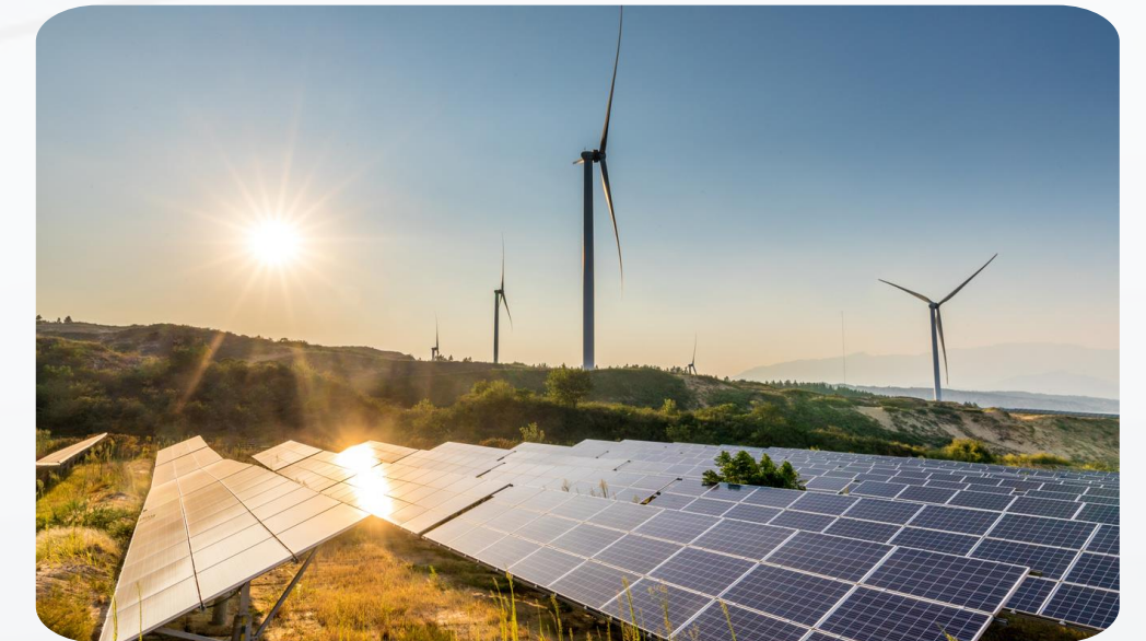
Wind power station at the Dnipro Water Treatment Plant - 2000 000 EUR
