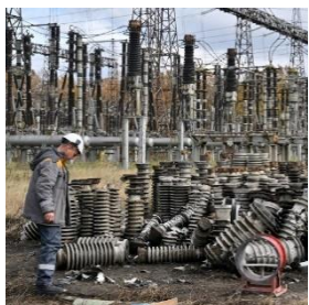
Energy (Infrastructure Rehabilitation)
