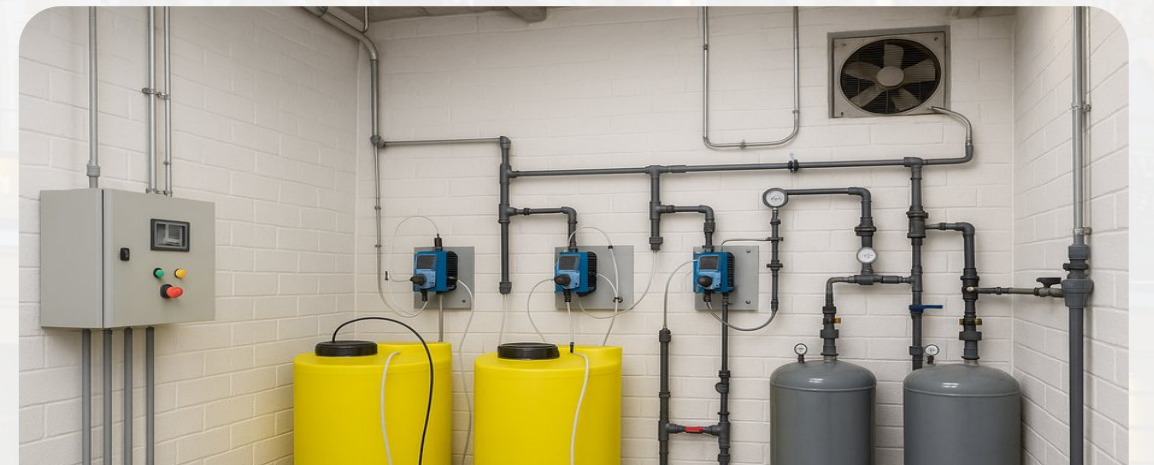
Reconstruction of the drinking water disinfection system using chlorine at the Dnipro water treatment plant 579 125 EUR
