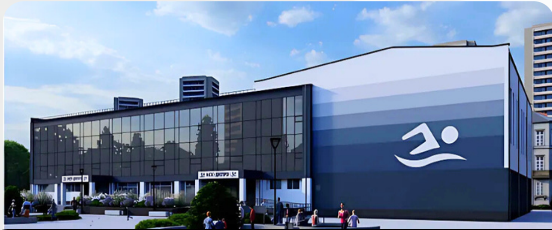
Major renovation of the sports and rehabilitation complex building with a swimming pool of the Municipal Enterprise «Municipal Sports Club «Dnipro» 1 500 000 EUR
