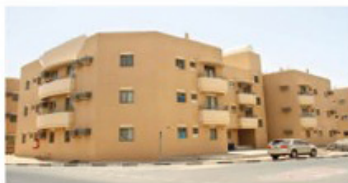
R327 F BLOCK BUILDING MUHAISNAH
