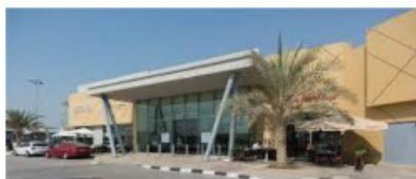
DISCOVERY GARDENS PAVILLION
