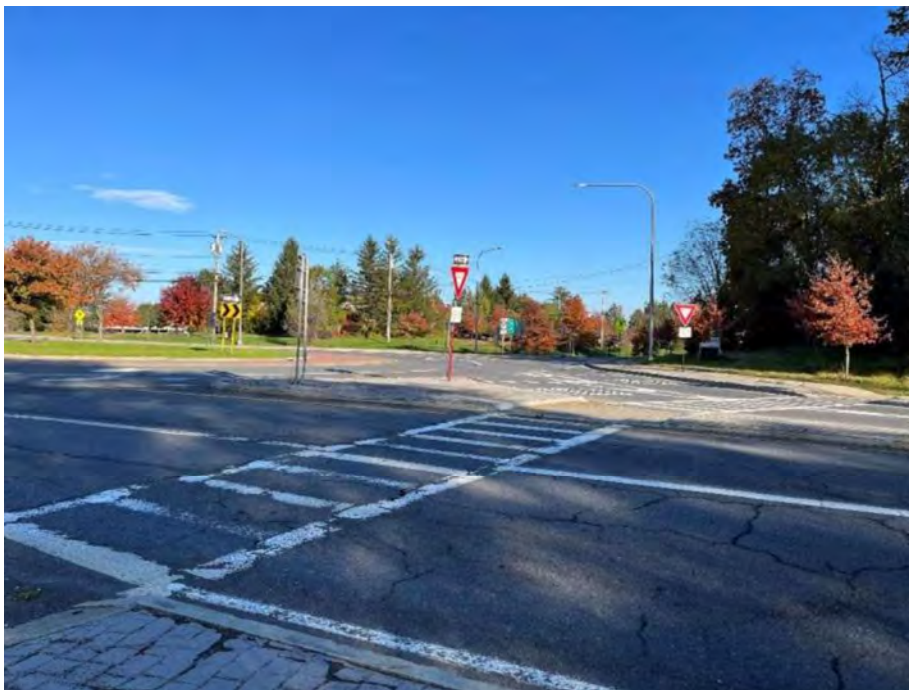
Photo 8: Looking north at the traffic circle.
