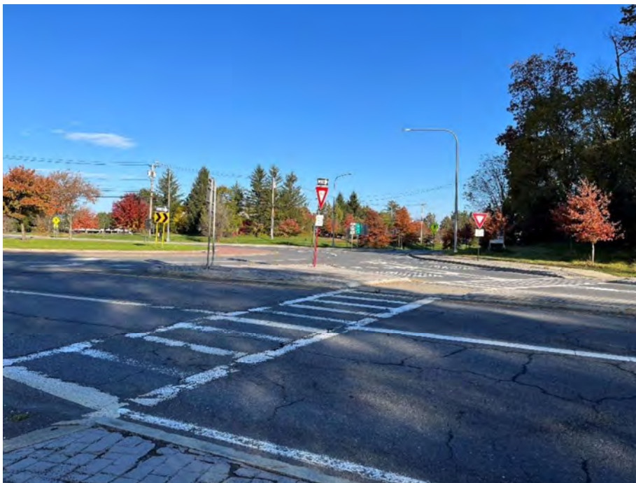
Photo 8: Looking north at the traffic circle.
