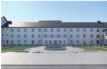
Reconstruction of a multidisciplinary hospital with the installation of a civil defence structure on the territory of the Irpin Central City Hospital
