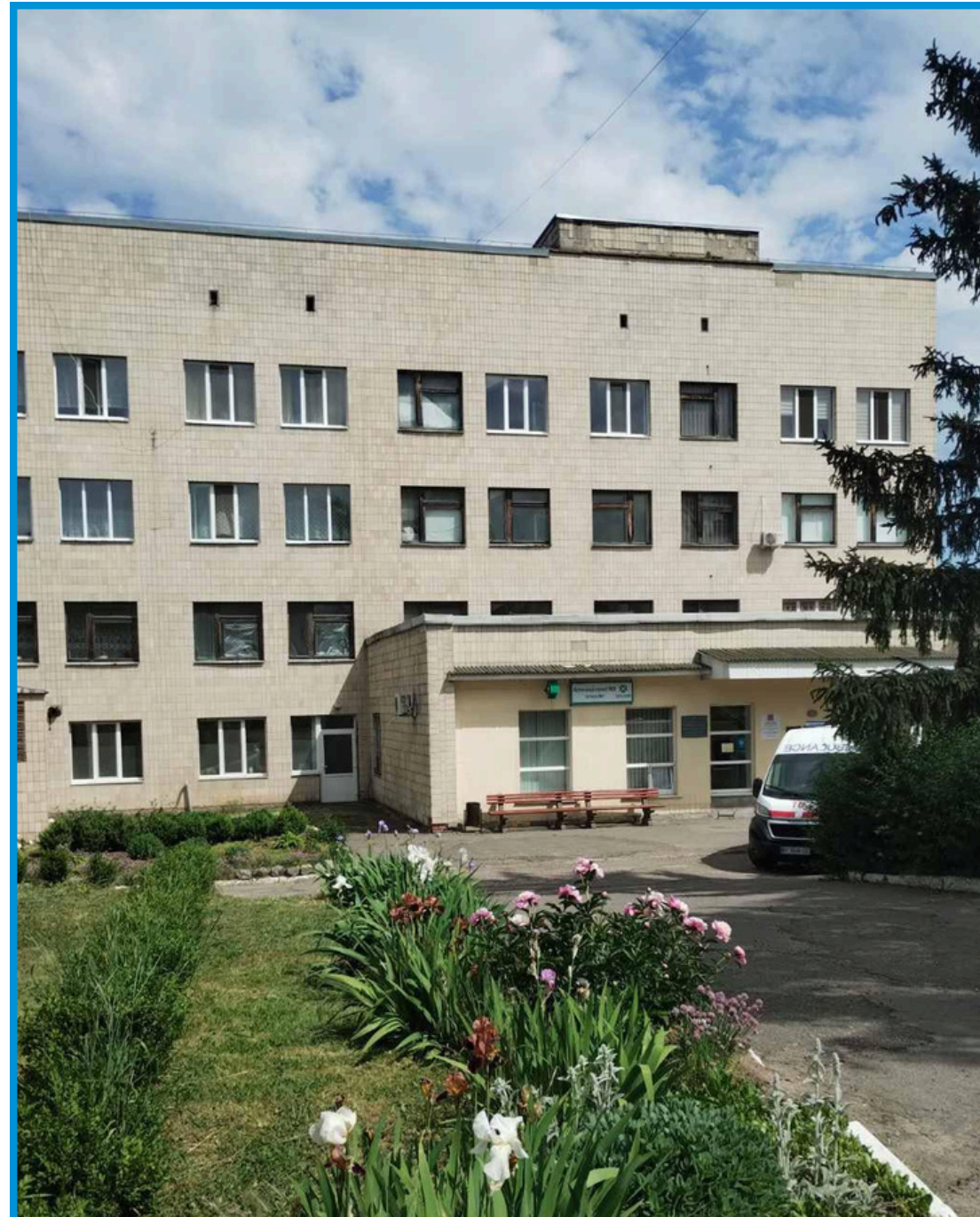
Reconstruction of the built-in premises of the building of the dental prosthesis laboratory and children's consultation in the rehabilitation department of the "Khorol City Hospital"
