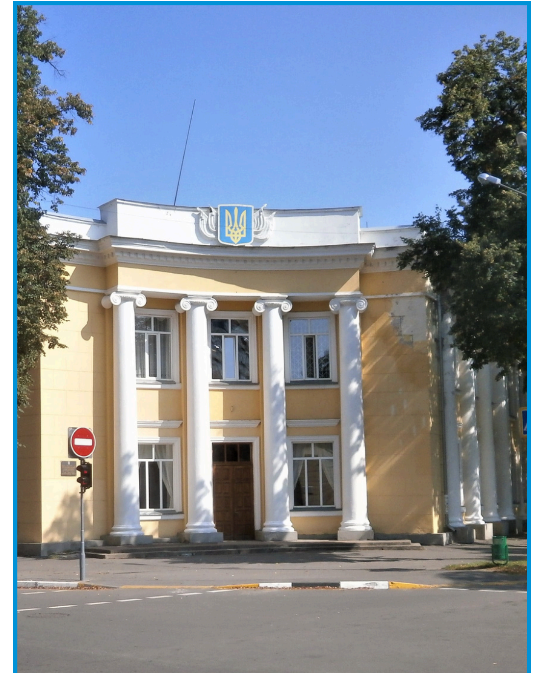
Restoration of the main building of the "Lubny Regional Hospital for War Veterans of Poltava Regional Council"
