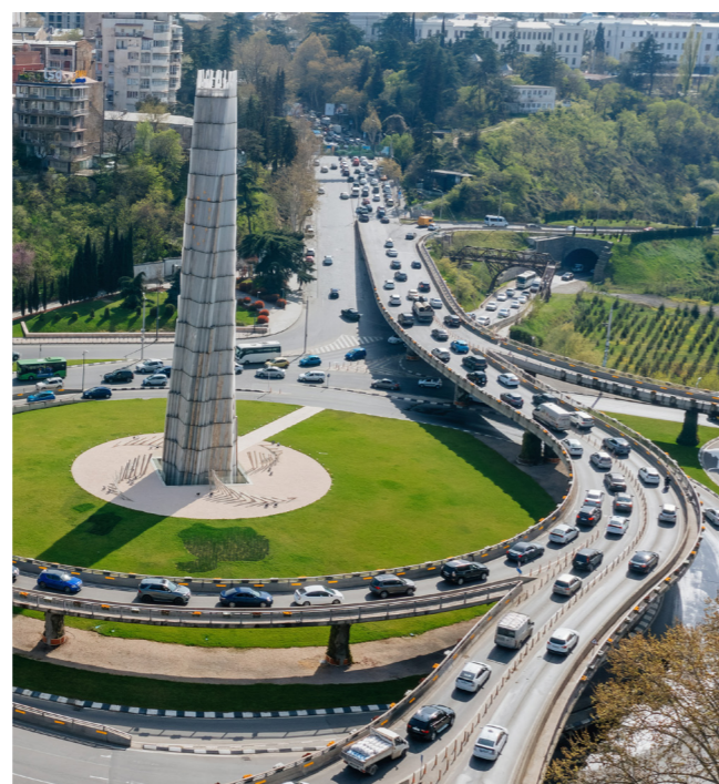
Ring Road junction near Square of Heroes Source: Mulderphoto - stock.adobe.com
