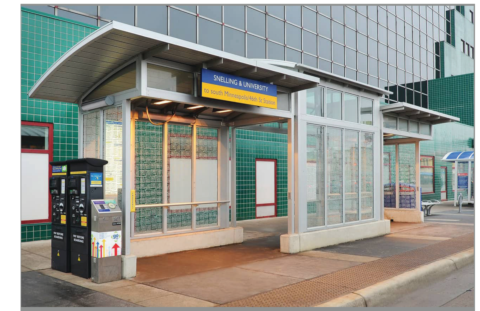
Metro Transit - BRT Station Source: Duo-Gard
