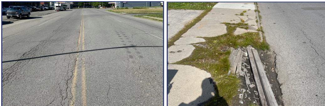
Figures 3, 4. Examples of non-compliant and deteriorating sidewalks and roadway conditions along Bailey Ave. These photographs were taken as part of a corridor-wide existing conditions assessment.
