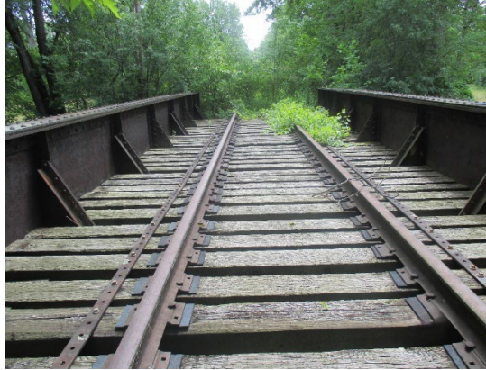
Bridge – Thru Girder
